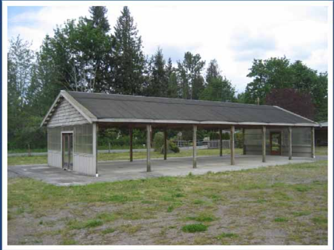
Pole Barn (Picnic) Shelter
